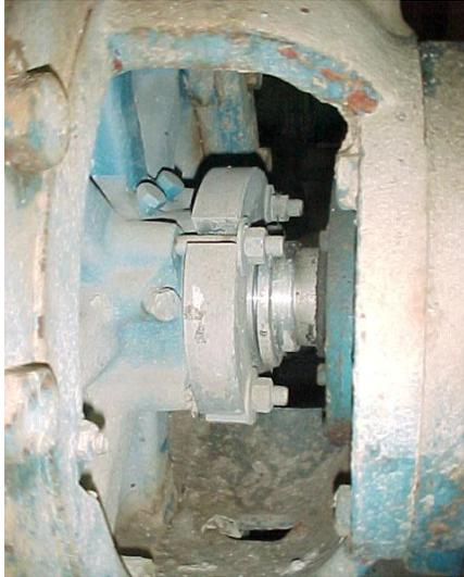
Huhnseal Diamond Seal still in operation; (installed in 1998).
